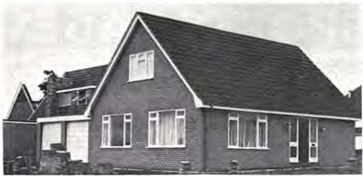
Another home ready, this time for Dave's son.
